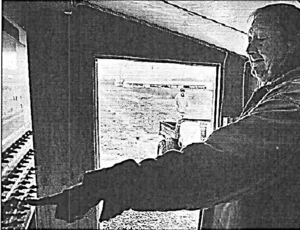
Dale Stevens checks the Rotem computer controller to his chickenhouses. The computer automatically governs the heat, ventilation and fans and relays the information to his home computer.
